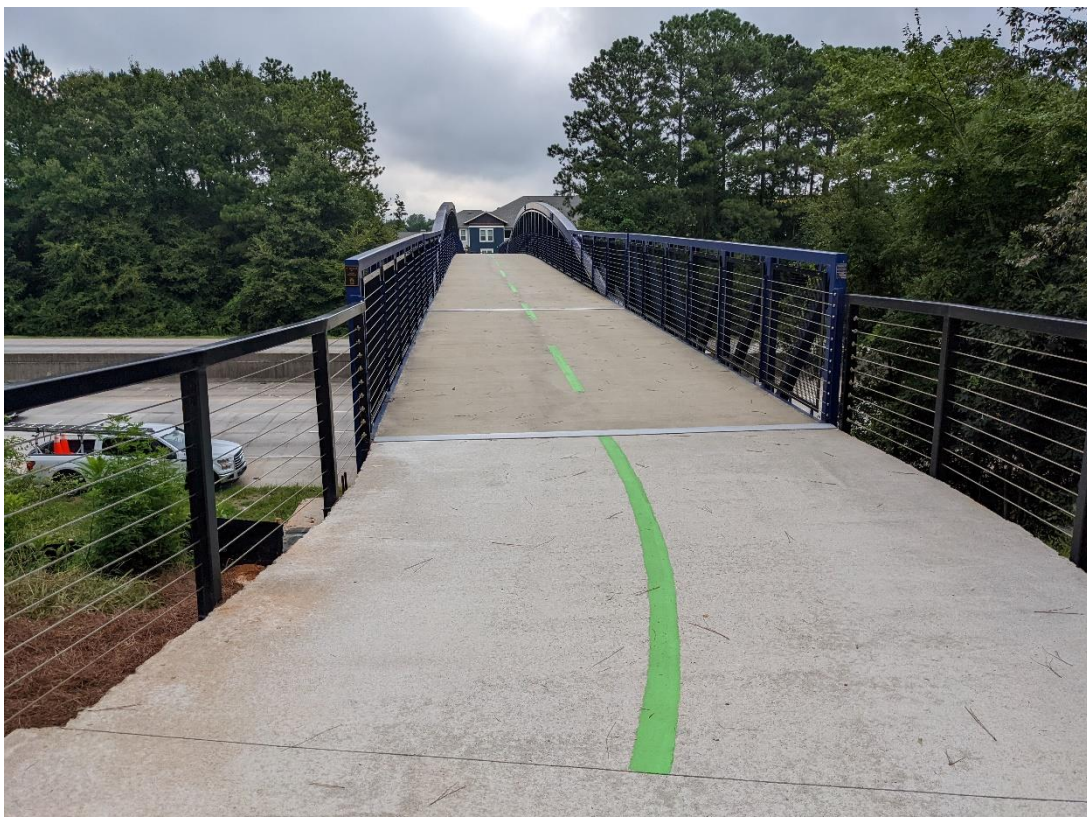
Photo 2 – Top of deck looking northeast. Direction of inventory.
